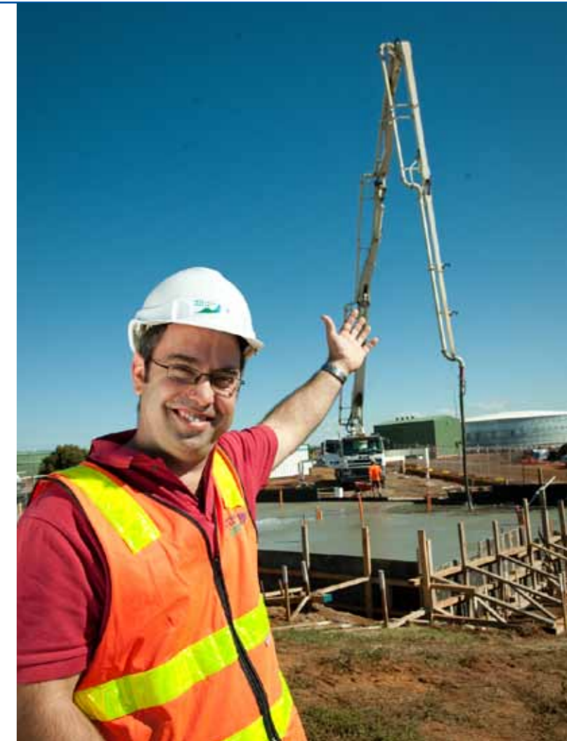
Western Water's Project Manager Justin Boan at the Cogeneration Plant construction site at Melton Recycled Water Plant before the launch.
