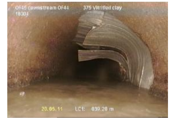
Non-standard Sewer works
