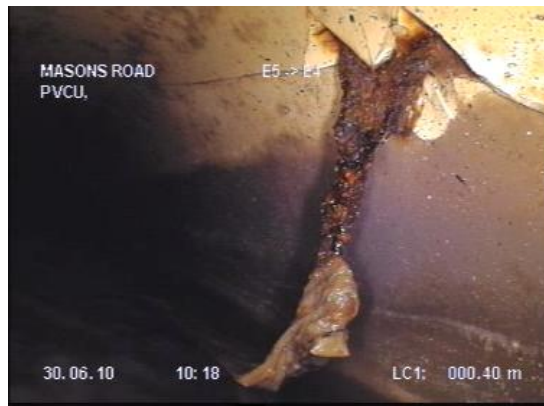
Object intrusions, (Fence posts, light poles etc)
