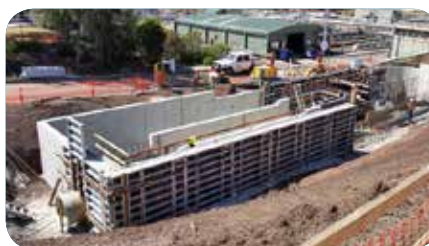
Testing of new membrane tanks (top). Construction of inlet works (above).
